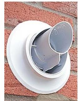
Flue terminal and air intake
